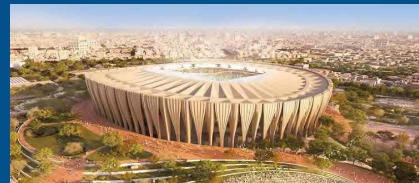
PRINCE FAISAL BIN FAHD SPORTS CITY STADIUM Riyadh
